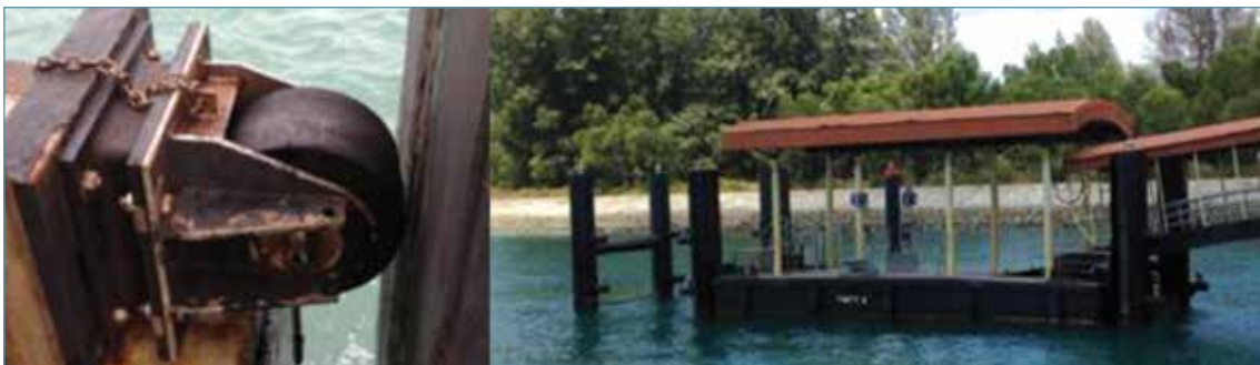
Existing roller, pontoon, and jetty berth at Tanah Merah Ferry Terminal
