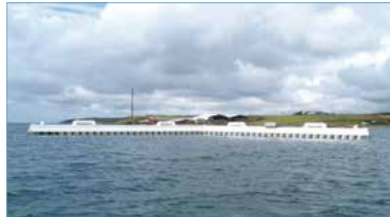
The 24 meter long Leancon system was installed in 2015 at the test site in Nissum Bredning
